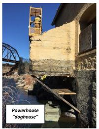
The overflow structure was balanced on wooden legs with no foundations and was perched on a 30-degree slope above an 80' cliff. Seismic requirements dictated that the new support system be constructed of structural steel. The steel supports required modern concrete footings constructed on an inaccessible rocky slope. Assumptions of bedrock conditions were made from visual inspection with the design to be finalized after the bedrock footings were excavated.
